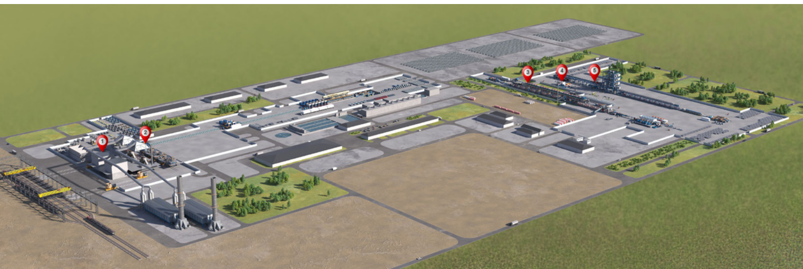
Design scheme of the new SDI Sinton flat roll steel complex: 1 – meltshop, 2 – CSP® plant, 3 – PL/TCM, 4 – skin-pass mill, 5 – galvanizing line (Picture: SMS group)
