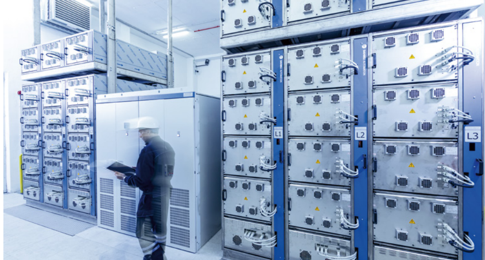
Figure 5. Q-ONE system with its installation was designed to ensure simple removal of the inverter and converter units, thus guaranteeing easy inspection and maintenance of the main components (Picture: Danieli)
