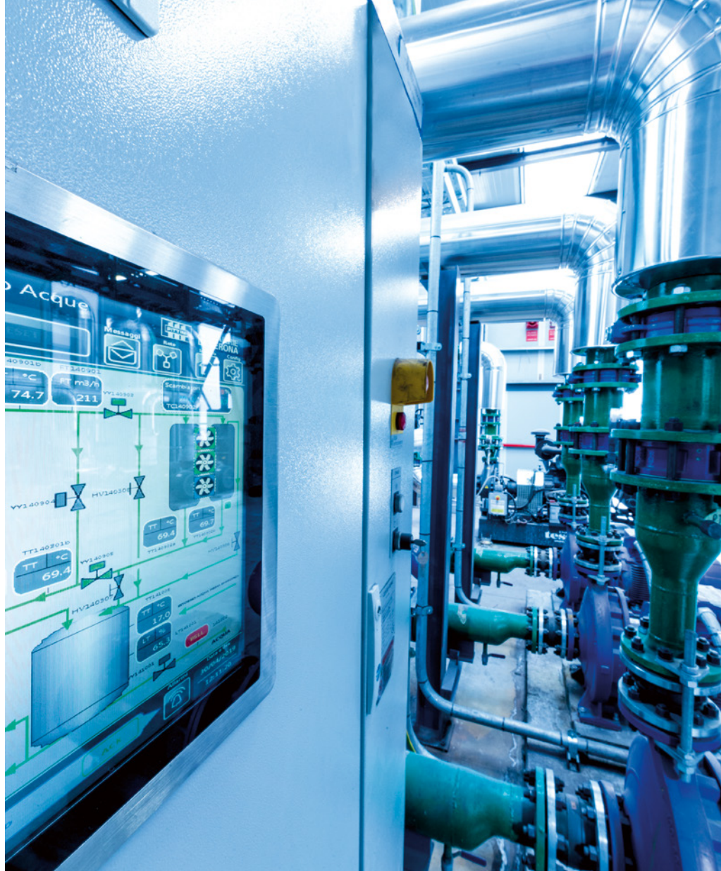
Figure 3. Pump room of the cooling water treatment circuit at Acciaierie di Verona (Pittini Group), which serves the Danieli FastCast six-strand billet caster and the two-strand wire rod mill with a 750,000-tpy capacity (Picture: Danieli)
