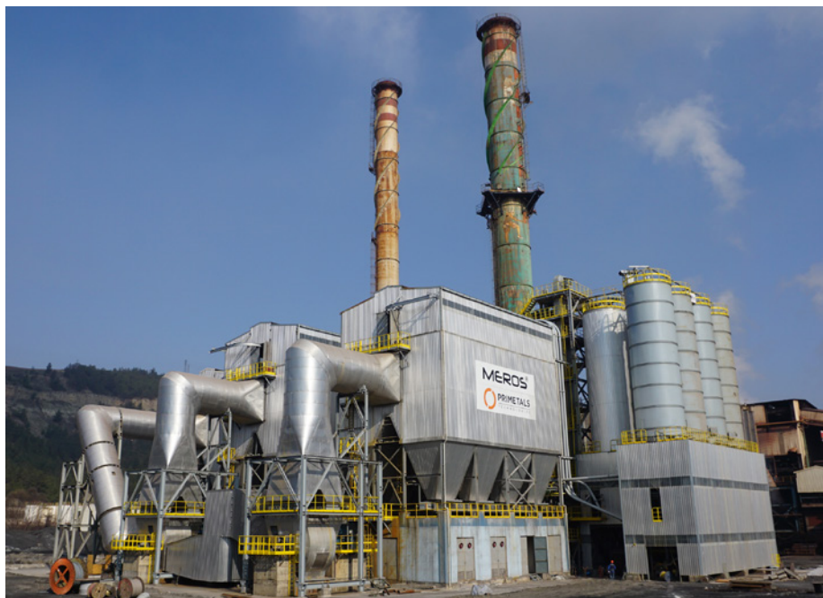
Off-gas cleaning plant at Karabük Demir Çelik Sanayi ve Ticaret A.Ş. (Kardemir) (Picture: Primetals Technologies)
