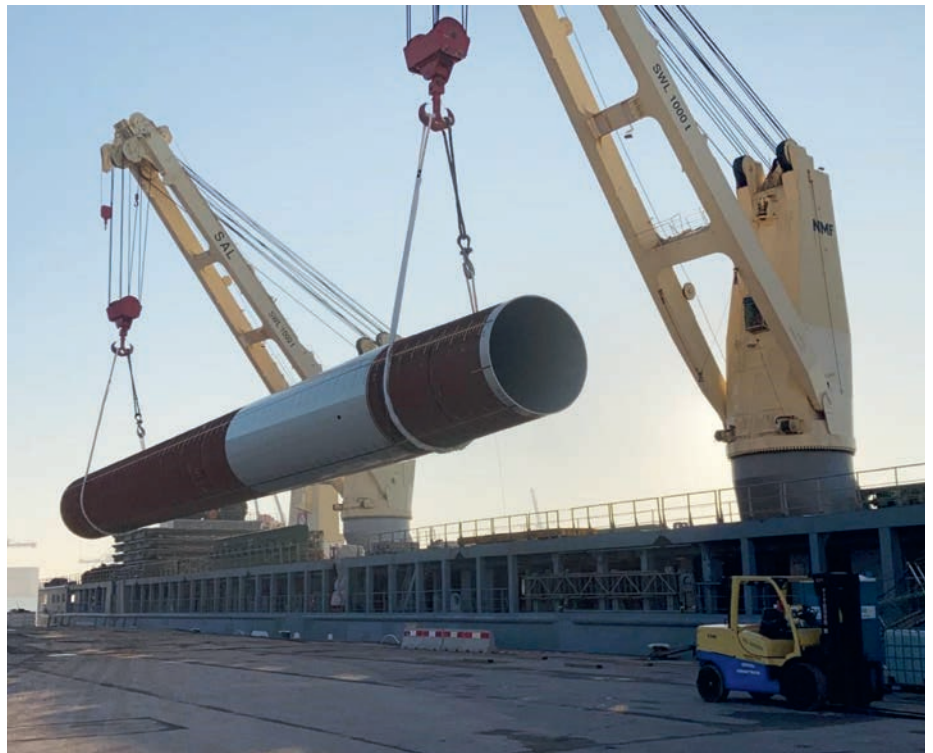
Unloading of the first monopiles for Akita Noshiro (Photo: Sif-Group)
