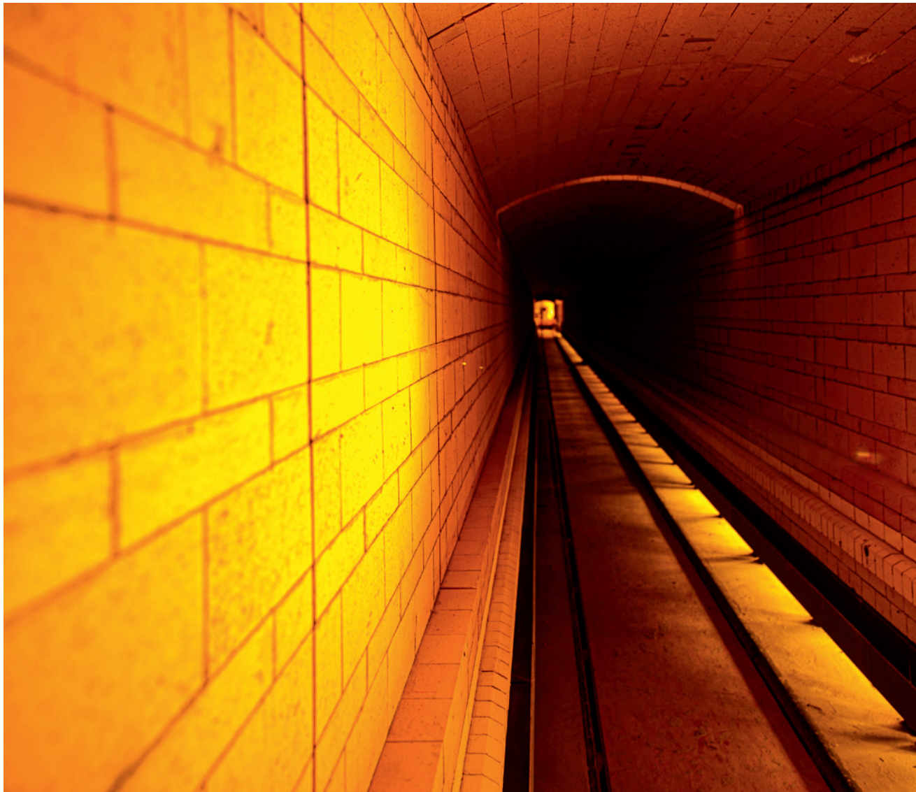
Photo: STEULER-KCH GmbH Refractory Linings
