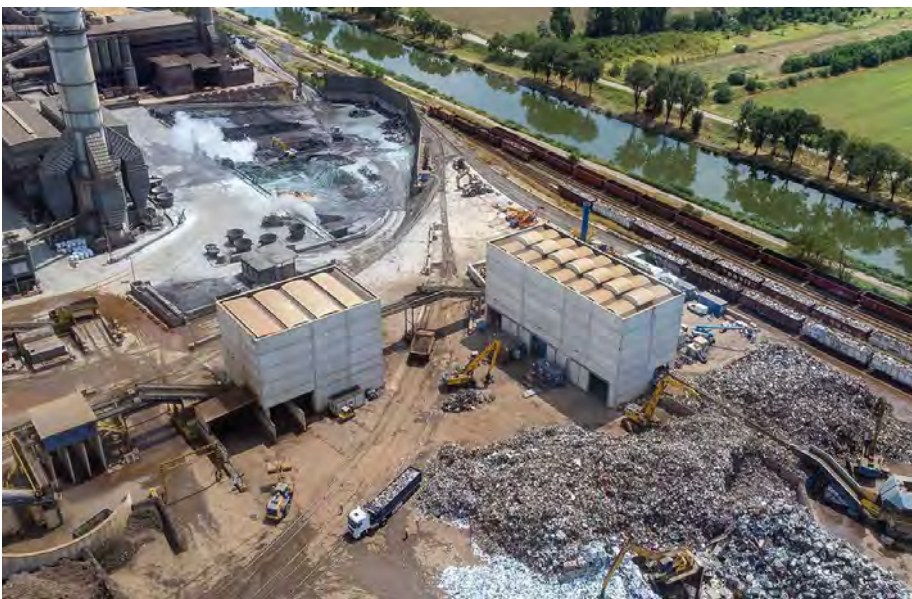
The new scrap processing plant at Acciaieria Arvedi in Cremona (Photo: Danieli)
