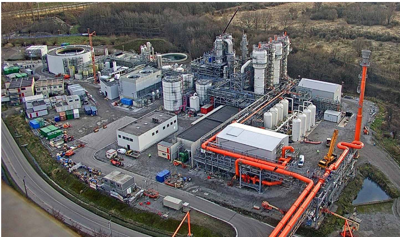
The gas is transported from the neighbouring steel plant via a large pipeline (orange) to feed the LanzaTech biocatalyst that convert this gas into ethanol (Picture: ArcelorMittal)
