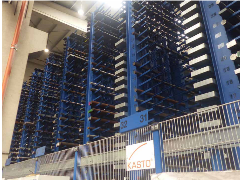
The new sawing centre at Bieber + Marburg has about 1,500 shelves and space for materials up to seven metres long and 330 millimetres in diameter (Picture: Kasto)
