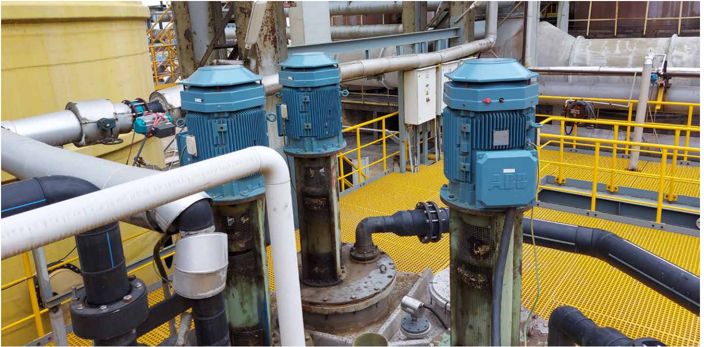
IE5 SynRM motors are ideal for rotating equipment like pumps, fans, and compressors distributed throughout the plant (Picture: ABB)
