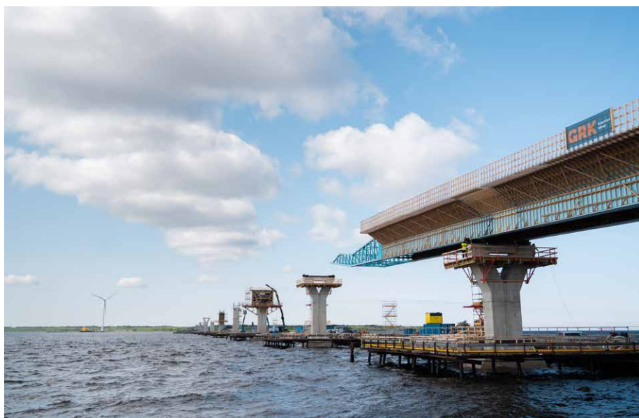
The bridge sections are huge: stand at over 4 metres in height, span 6 metres in width, and extend 26–32 metres in length (Picture: SSAB)
