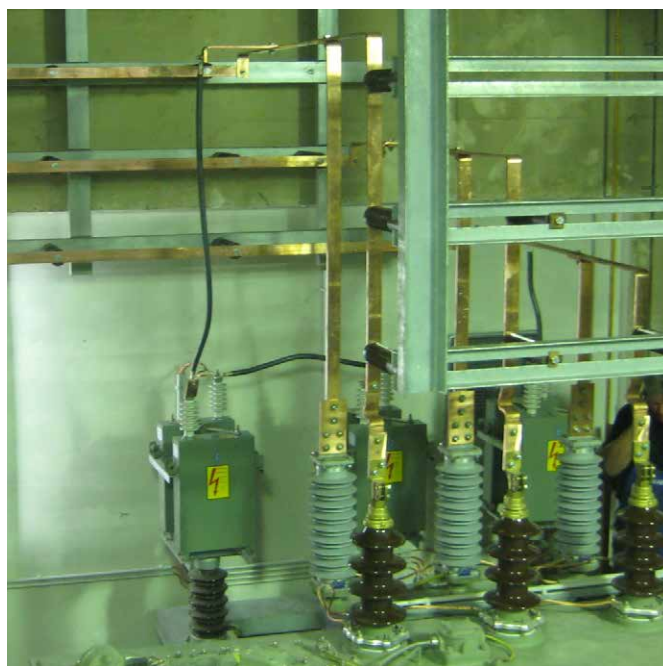
Figure 4. RC filters and surge arresters close to transformer HV terminals, copper busbars to VCB switchgear (Picture: BSE)
