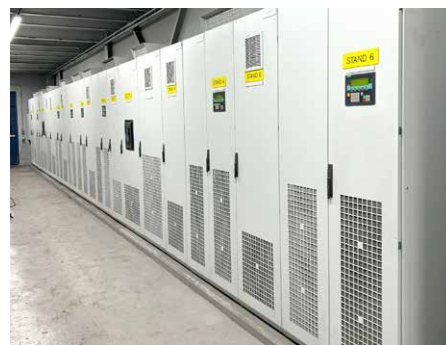
Sterling Steel's rolling mill now operates with 16 upgraded DC drives (Photo: Primetals Technologies)
