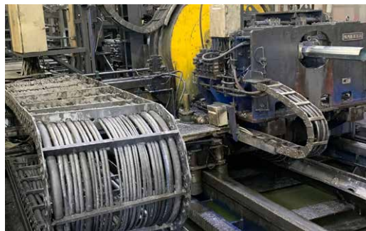
Upgraded automation and drives system for a 12-inch Nakata flying cutoff machine (Picture: Primetals Technologies)
