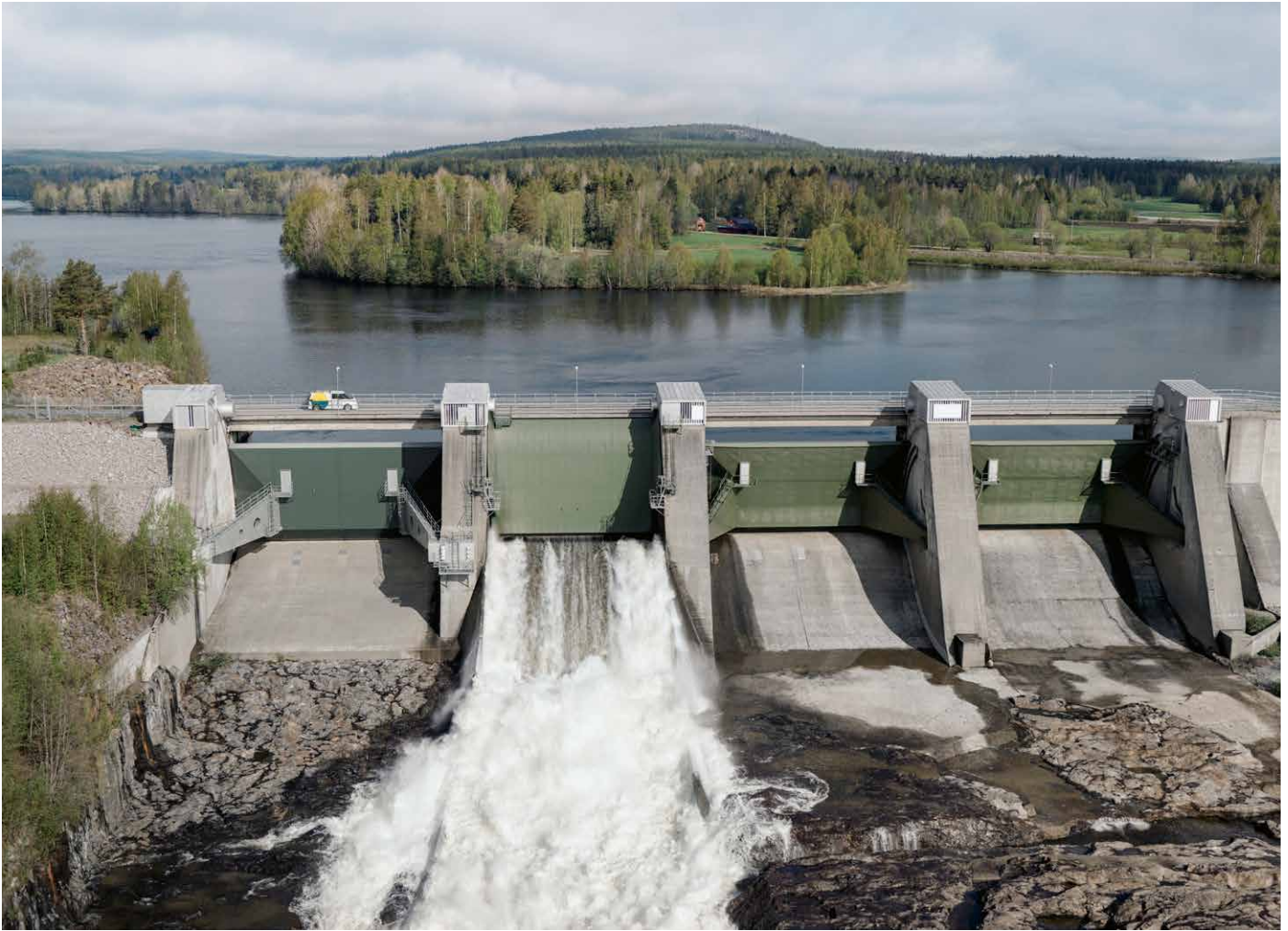
Stornorrfors dam on the Ume River in Sweden (Picture: Vattenfall)
