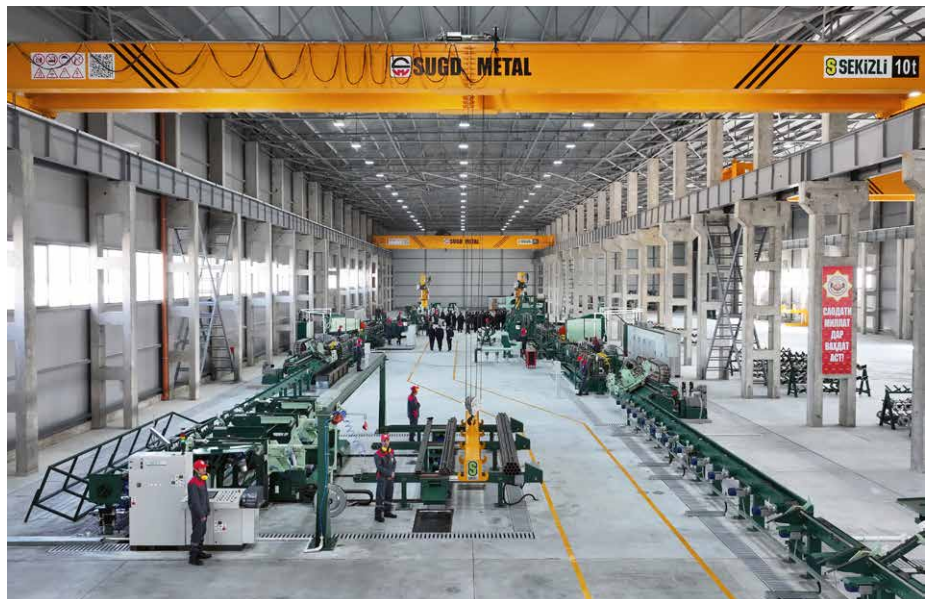
General view of the tube production facility at Sughd Metal (Picture: Fives)
