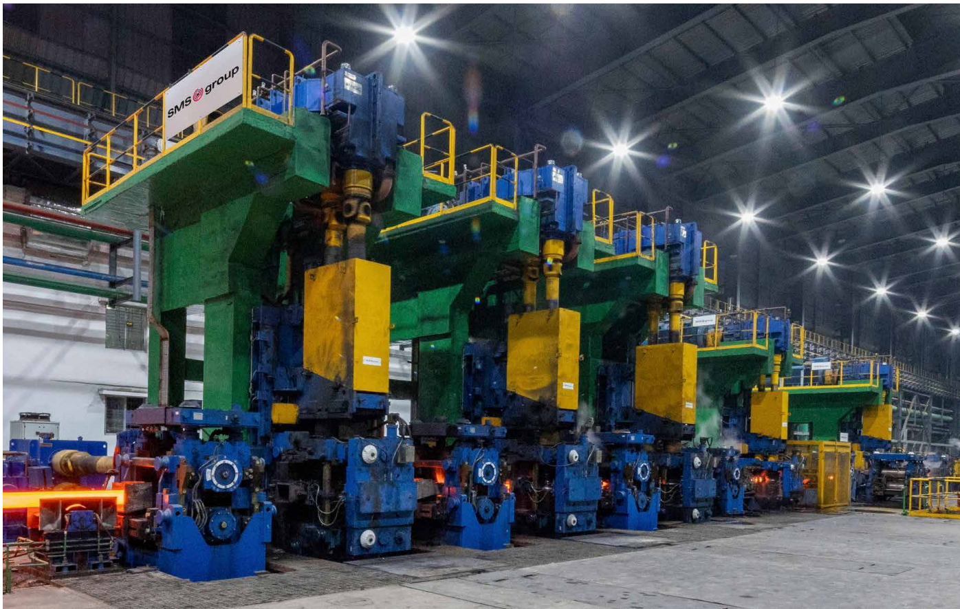
The rebar mill achieved a speed of 55.04 meters per second for the production of 2x10-millimeter deformed bars (Picture: SMS group)
