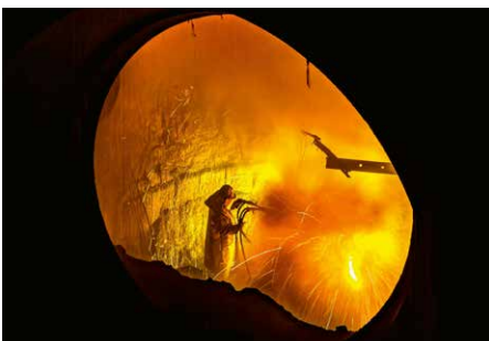
Repair work inside the blast furnace (Photo: SMS group)
