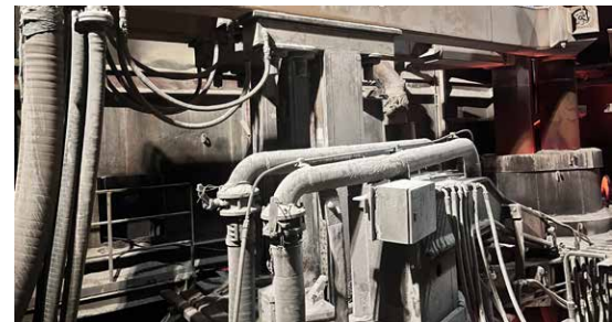
New electrode arms boost power output and reduce energy consumption at Tonghua Iron and Steel
