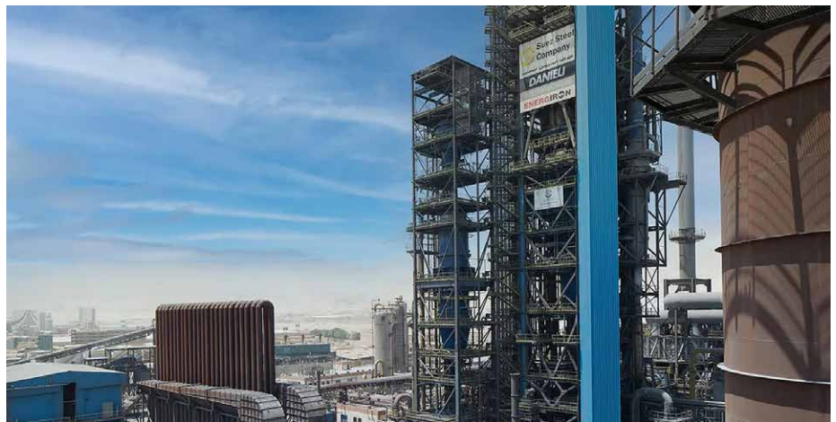
Suez Steel has reached natural gas consumption levels slightly below 2.2 Gcal per tonne of DRI produced (Picture: Danieli)
