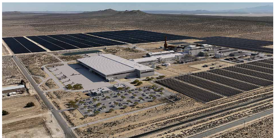
The new EAF steel plant built by Pacific Steel Group in Mojave, California (Photo: PSG)
