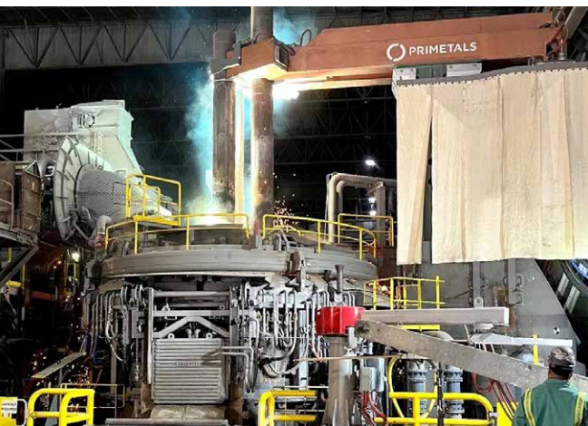
The first heat for NLMK Indiana's 118-ton EAF after the modernization
