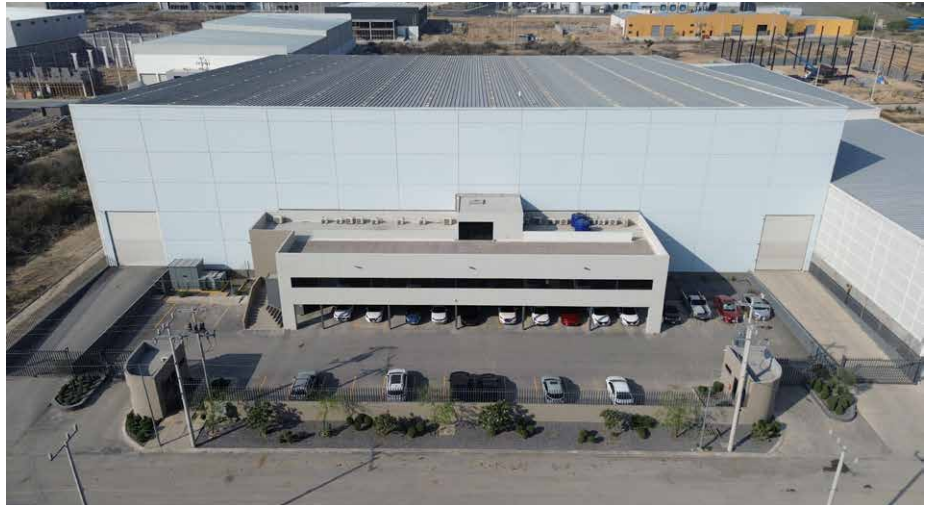
The facilities of Aceroteca Trading located in Santa Catarina within the metropolitan area of Monterrey, Nuevo León, Mexico (Picture: thyssenkrupp Material Services / Aceroteca Trading)
