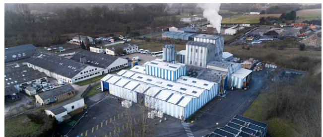
The production site of Calderys in Abbeville, France (Picture: Olivier Lattuga-Duyck for Calderys)
