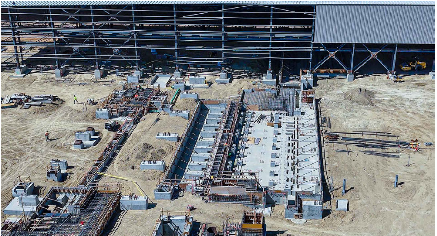
Pacific Steel Group is building California's first new steel mill in more than 50 years, with commissioning scheduled for 2027 (Picture: Danieli)
