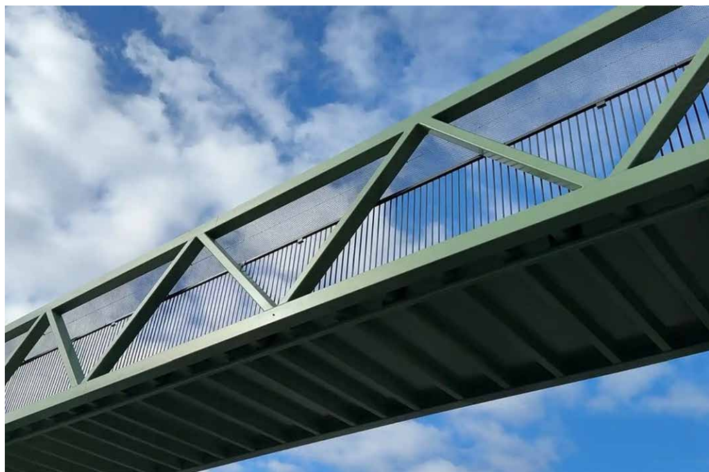
The first bridge built using decarbonized steel spans the E22 highway in Lund, Sweden. (Picture: SSAB)
